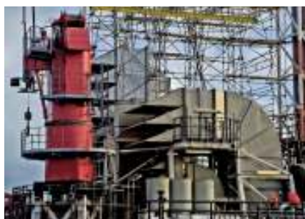
Installation of AAF low velocity system, original high velocity system in the foreground
