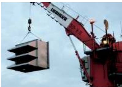
Installation of AAF low velocity system
