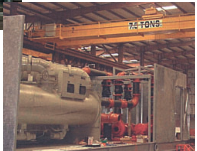
Efficient McQuay centrifugal chiller with interconnecting pipes, valves, and wiring.
