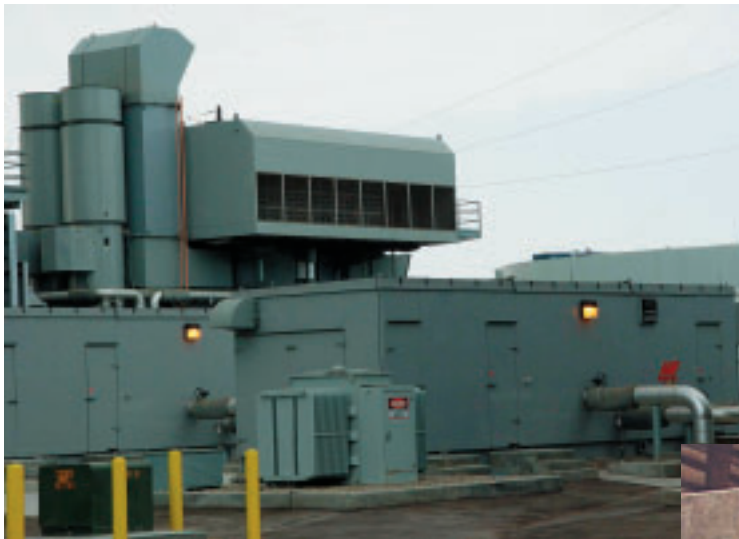
An AAF packaged chiller cools inlet air for GE LM6000 gas turbines at a California utility.
