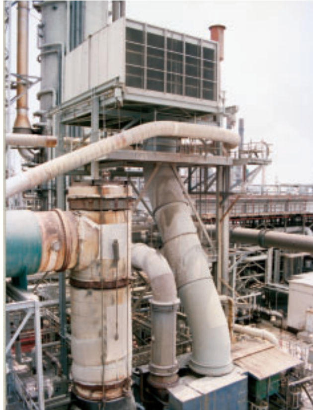
AAF supplied a retrofit inlet air system with evaporative cooling for a compressor at a refinery in LA.
