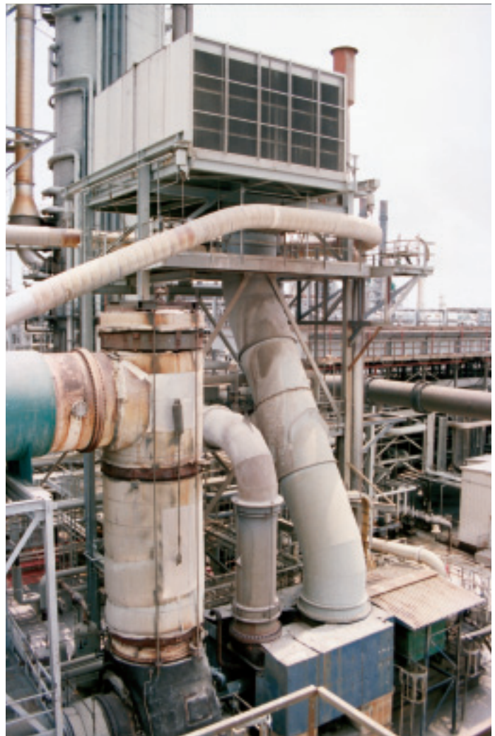
AAF supplied a retrofit air intake package with evaporative cooling for a FCC compressor at a BP refinery at Belle Chasse, Louisiana.
