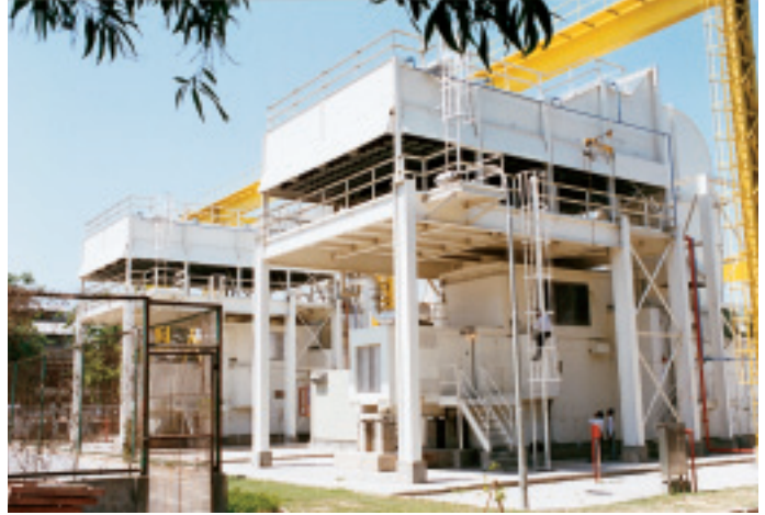
AAF supplied a Pulse Jet filter for a Westinghouse W-251 turbine at Bali, Indonesia.
