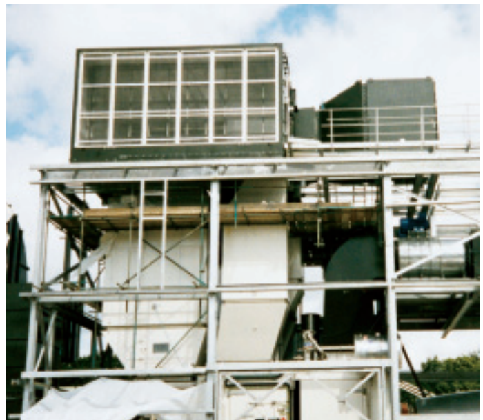
AAF supplied a retrofit air intake package with evaporative cooling for a FCC compressor at a BP refinery at Belle Chasse, Louisiana.
