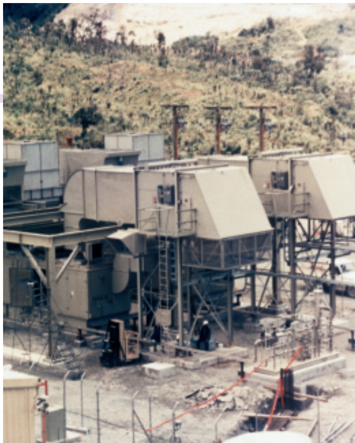
AAF supplied air intake and exhaust systems for a Solar Mars Turbine at Placer Dome, New Guinea.
