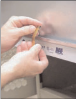
Remove front prefilter clip
