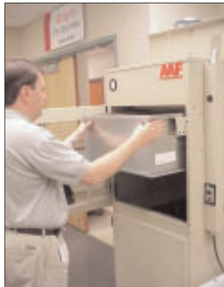
Slide filter onto top of filter support frames. Make sure locking levers are pushed all the way in to the unit or damage to the HEPA seal could occur.
