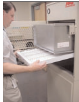
Insert prefilter into rear clip
