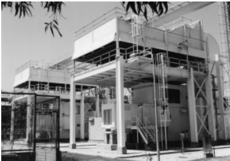
AAF Pulstar inlet filtration system for two Westinghouse W-251 turbines located in Bali, Indonesia.
