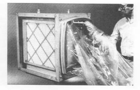
Withdraw the prefilter into the bag by sliding it along its mounting track. Some enclosure styles include filter removal rods to assist with filter removal on multiple filter wide enclosures. The filters are drawn towards the access door by pulling on the removal rod. Ensure that the bag/collar connection remains secure during this operation.
