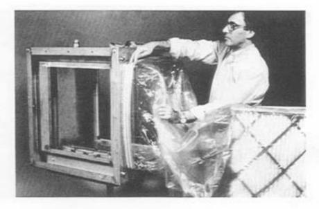
Insert the replacement filters into a new bag and, with the old bag stub still in place, install the elastic cord of the new bag onto the vacated inner groove of the Bag-In/Bag-Out enclosure collar.
