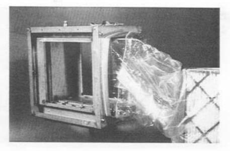
Replace the security strap on the new bag and tighten it down firmly. The new filters may now be installed.
