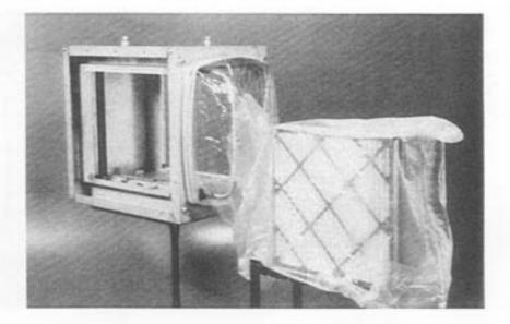
In preparation for sealing the bag move the filters away from the door opening to extend the bag. As always, ensure that the integrity of the bag/collar connection is maintained.
