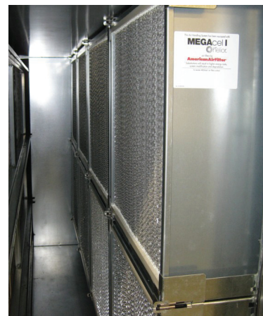
MEGAcel I filters installed in Cancer Treatment Centers of America
